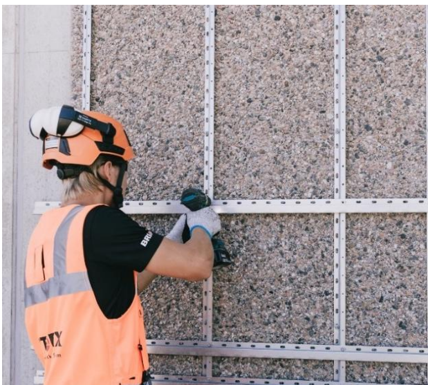
Picture 24: Installation of mounting rails
