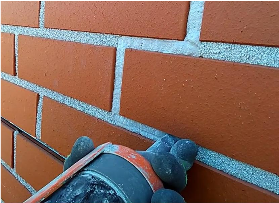
Picture 41: On-site jointing
