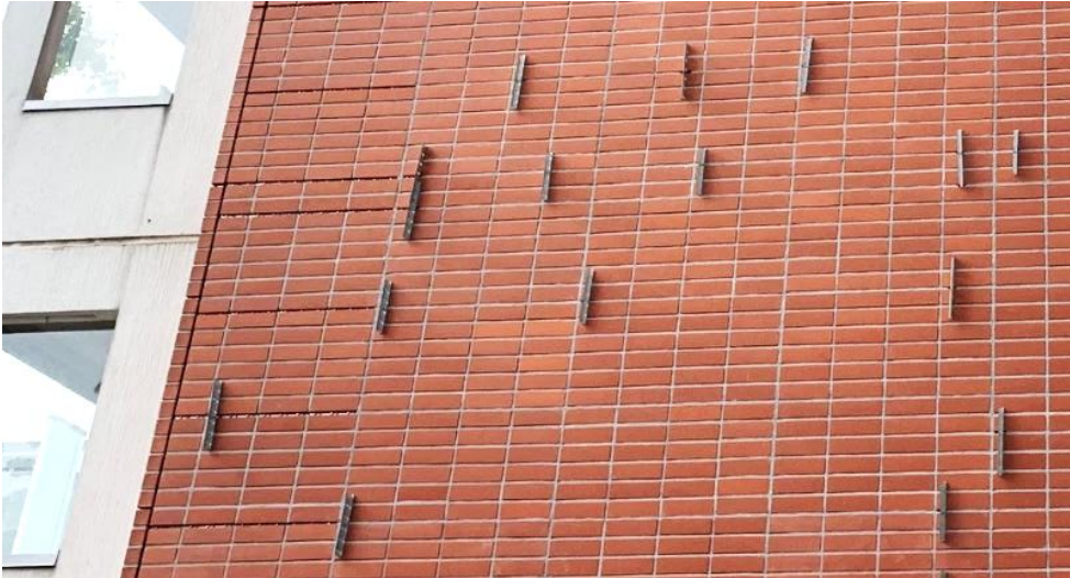
Picture 34: The evenness of the brick surface is ensured before the jointing
