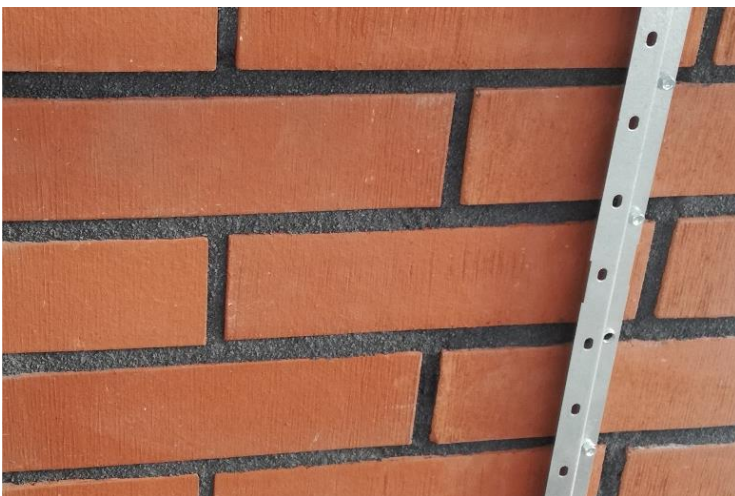
Picture 37: Support rail for brick slip being replaced
